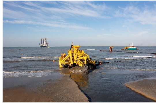
Figure 2-10 Vessel fed jetting
