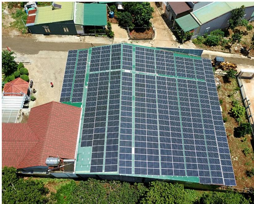
Figure 45: PV solar rooftop in Dak Nong province (135 kWp)
