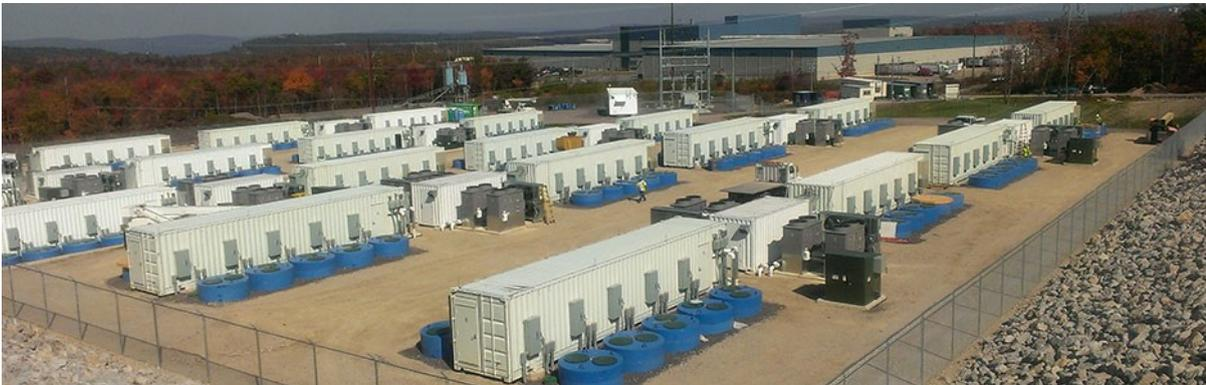
Figure 32: Photo of Beacon Power flywheel installation in commercial operation in PJM, Hazle, Pennsylvania. The plant includes 200 flywheel modules lowered into the ground (5 on each side of a container). The plant currently provides 20 MW of frequency regulation service to PJM and reached full commercial operation in July 2014 [6].
