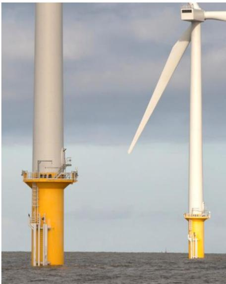
**Figure 3-11 Photo of typical wind turbine in operation with monopile foundation**
