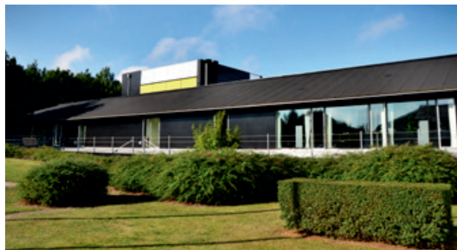
Rockwool International office building was recently renovated to upgrade energy performance. The building envelope was improved with new and better insulated façades and new windows. Also, heat collectors and PV has been installed on the roof for energy production. (Photo: ROCKWOOL)
