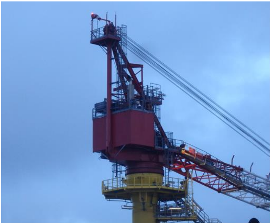
Figure 62. Instruments position on Harald B oil rig. Source: Total Energies.
