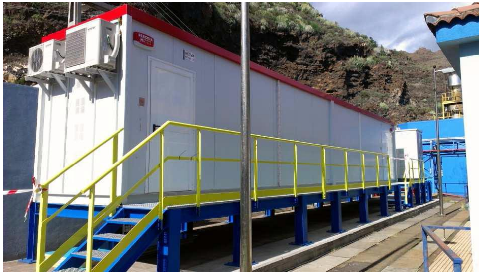
Figure 2.51. La Palma supercapacitor. Source: (Mahmoudi, Chaffour, Goosen, & Bundschuh, 2017)
