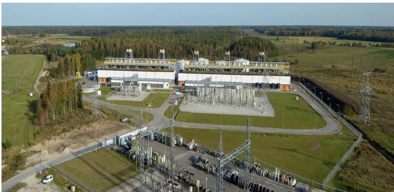
Figure 3 Kiisa emergency reserve power plant (ERPP) in Estonia [14].
