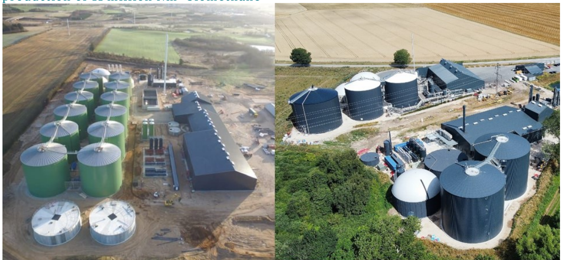
Figure 4: SBS Kliplev (left) is approx. 8.5 ha and has an annual production of 48 million Nm 3 of biomethane, whereas Solrød Biogas (right) is approx. 2 ha and has an annual production of 11 million Nm 3 biomethane
