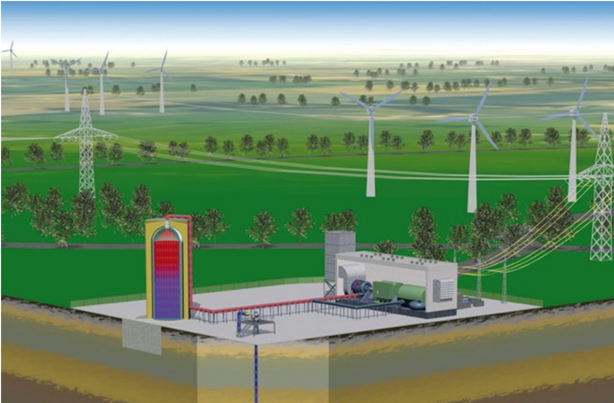
Figure 7: RWE's vision for an ACAES plant [15].
