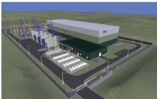
Figure 4. Example of layout of HVDC, VSC substation, Greenlink 6 [50].
