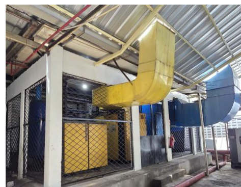
Figure 26 : Installed hot air exhaust for compressor
