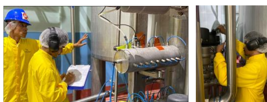
Figure 21 : Air leakage detection point in tubing and pneumatic actuator
