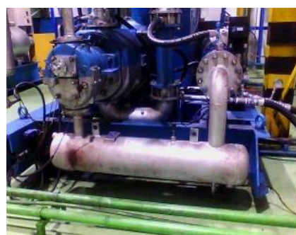
Figure 30 : Hot compressed air at point of 3 stage compressor
