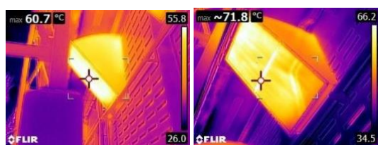
Figure 27 : Exhaust hot air after cooling fan discharged to the atmosphere
