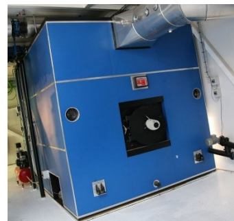
Figure 21: 250 kW pellet boiler for large buildings from LIN-KA [16]
