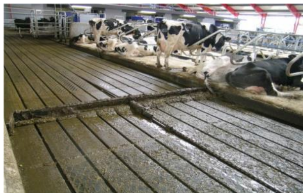
Figure 4. Cubicle barn with precast concrete solid drained floor in the walking alleys. (Photo: Perstrup A/S).
