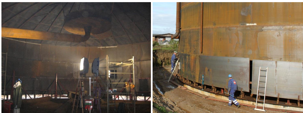
Figure 4: Left: Top diffuser in a 5,500 m 3 TTES under construction in Brædstrup, DK. Right: 5,500 m 3 TTES under construction. The tank is lifted and welded from beneath. Photo: Brædstrup Fjernvarme.
