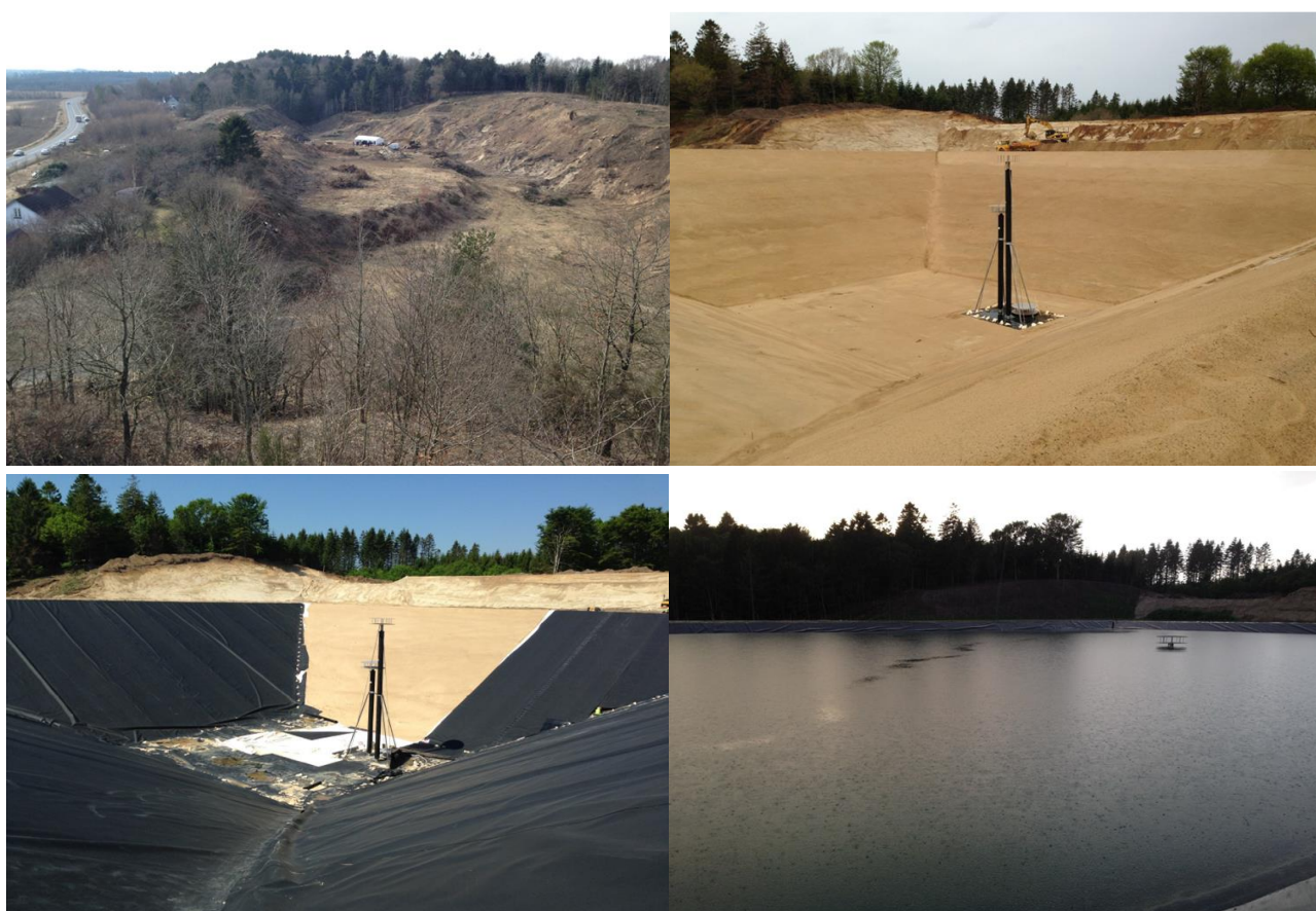
Figure 7: Upper left the abandoned gravel pit. Upper right excavation is finalized, and the in- and outlet is implemented. Bottom left HDPE membrane is mounted. Bottom right water has been filled in. Photos: Dronninglund Fjernvarme.
