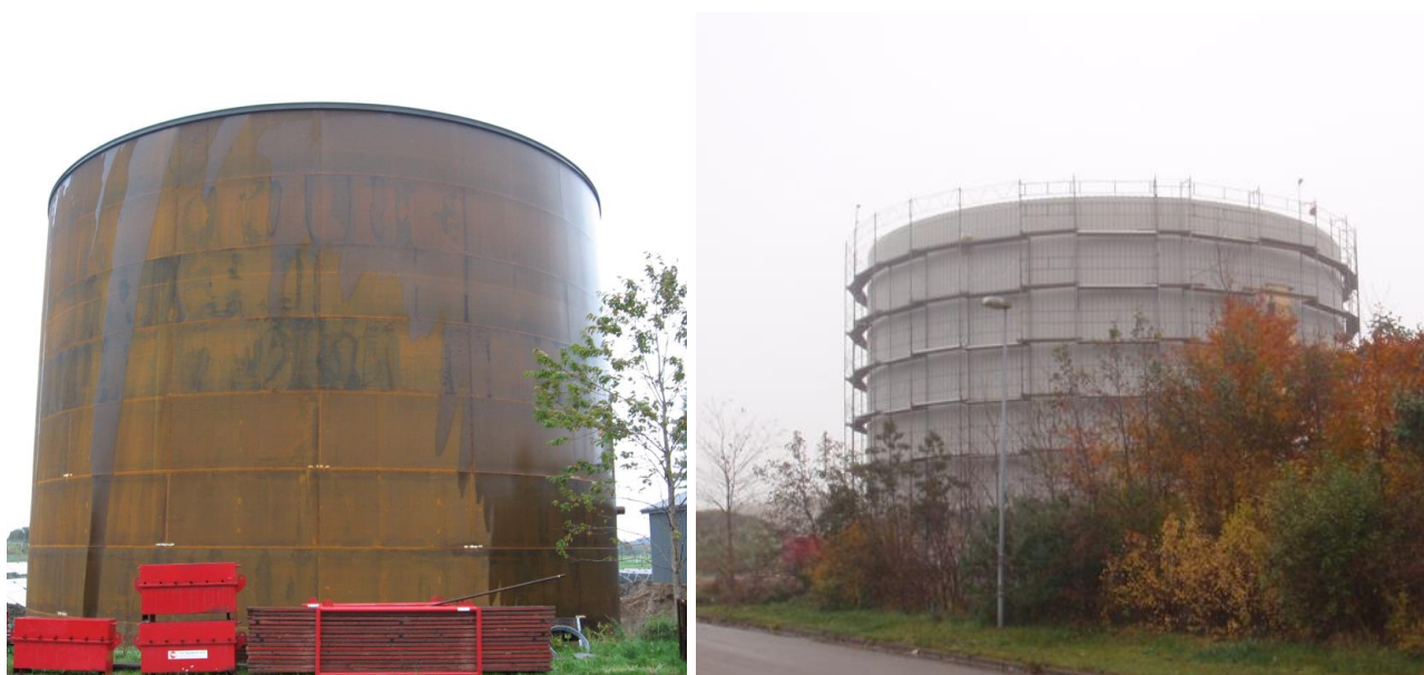
Figure 5: Left: 5,500 m 3 TTES finalized without insulation. Right: Insulation and covering finalized.
