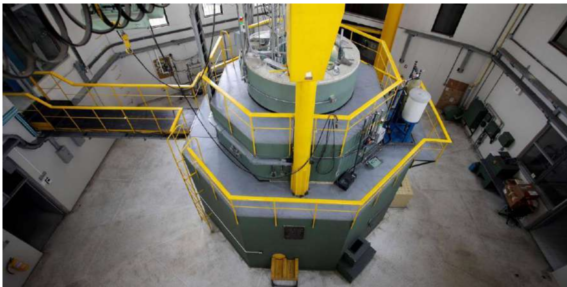
Figure 113. IAN-R1 Reactor at the Colombian Geological Service [32].
