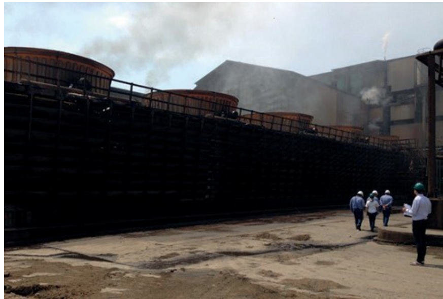
Figure 14: Cooling tower from Mexican sugar mill
