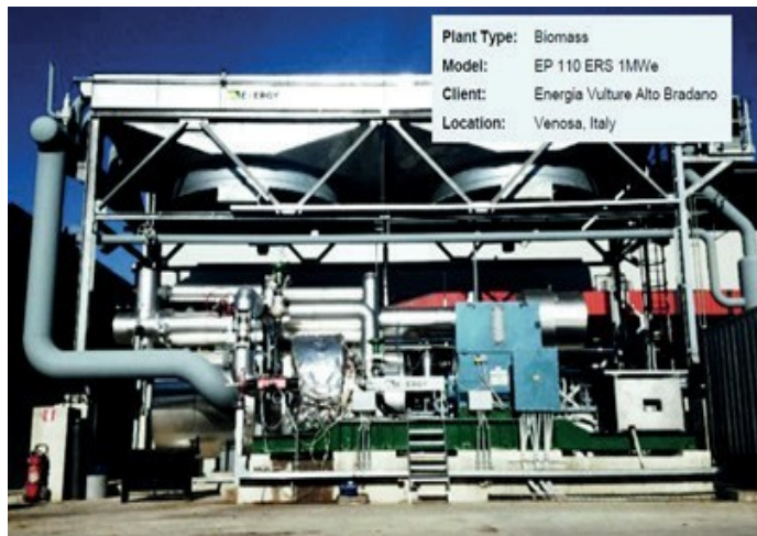
Figure 19: A 1 MWe biomass driven ORC unit [4]
