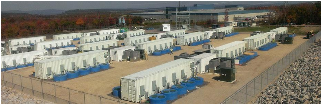
Figure 2.54. Hazle Township, Pennsylvania. Source: (DTU Energy, 2019)
