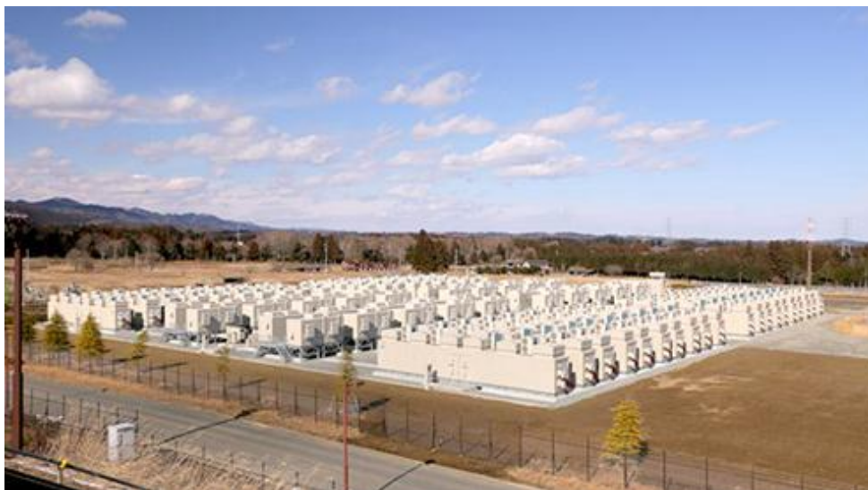
Figure 2.16. Minima-Soma storage system of Tohoku Electric Power Company. Source: (Toshiba, 2016)
