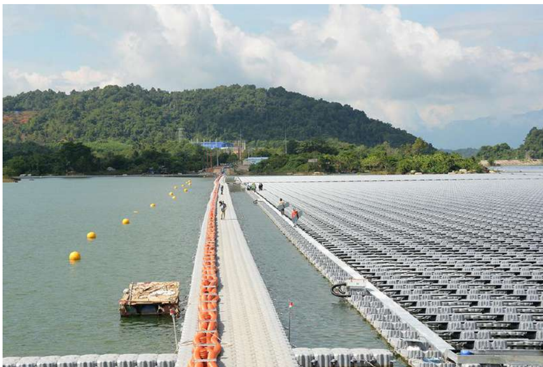
Figure 48: Da Mi solar power plant – 47.5 MW p
