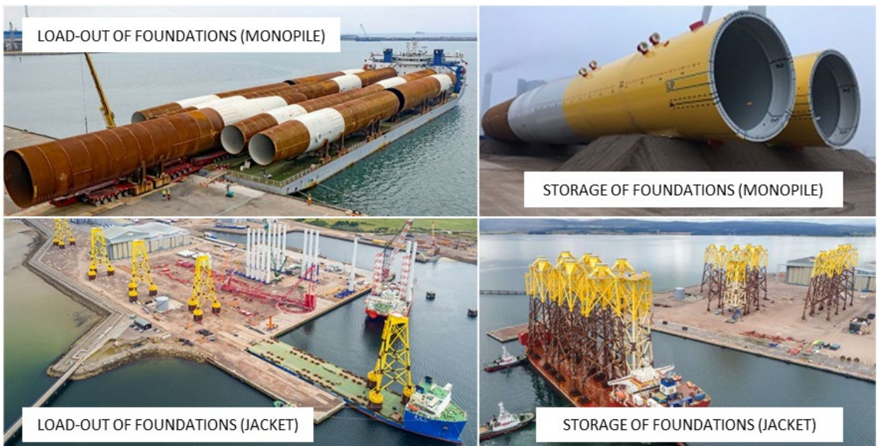
Figure 5-5: Typical loadout and storage operations for foundations
