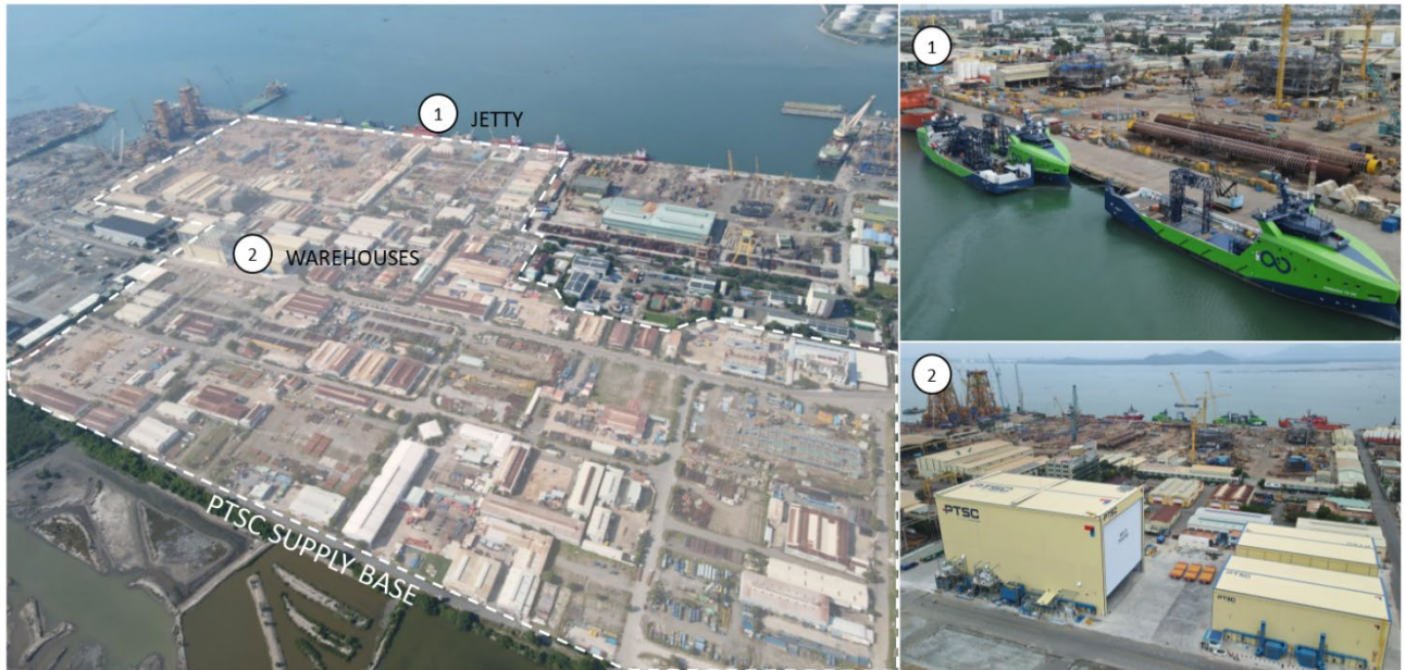
Figure 7-3: PTSC Supply Base - Vung Tau
