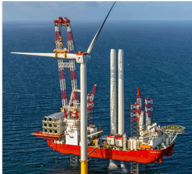
Figure 7-8: Typical Wind Turbine Installation (WTIV) - PTSC Downstream
