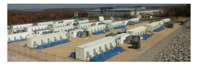
Figure 5: Photo of Beacon Power flywheel installation in commercial operation in PJM, Hazle, Pensylvania. The plant includes 200 flywheel modules lowered into the ground (5 on each side of a container. The plant currently provides 20 MW of frequency regulation service to PJM and reached full commercial operation in July 2014 [6].
