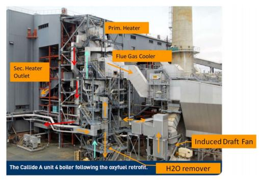
Figure iii-10 Photo of Callide Oxy-fuel boiler from [52] showing retrofit paths (red) and flue gas flue directions (yellow).
