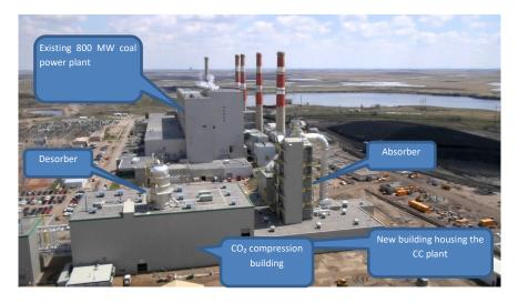
Figure ii-4. Photo [59] of Saskpower 800 MW<sub>e</sub> Boundary Dam coal-fired power station where one of the four units was retrofitted with amine CC in 2013.
