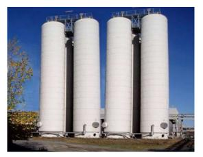
Figure 9. Storage for 3300 tons liquid CO<sub>2</sub> at Yara's ammonia plant in Porsgrunn, Norway in conjunction with CO<sub>2</sub> export terminal (now operated by Nippon Gases Norway) [7]
