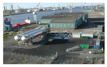
Figure 10. Liquid CO<sub>2</sub> import terminal with truck filling bays operated by Yara (now Nippon Gases Norway). [7]
