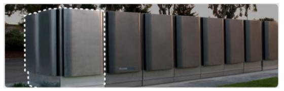
Figure 4: BloomEnergy SOFC system. The dashed region corresponds to ine 250  $kW_{\rm e}$  unit [1].
