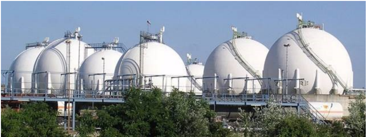
Figure 0-29: Typical gas storage tanks [21]
