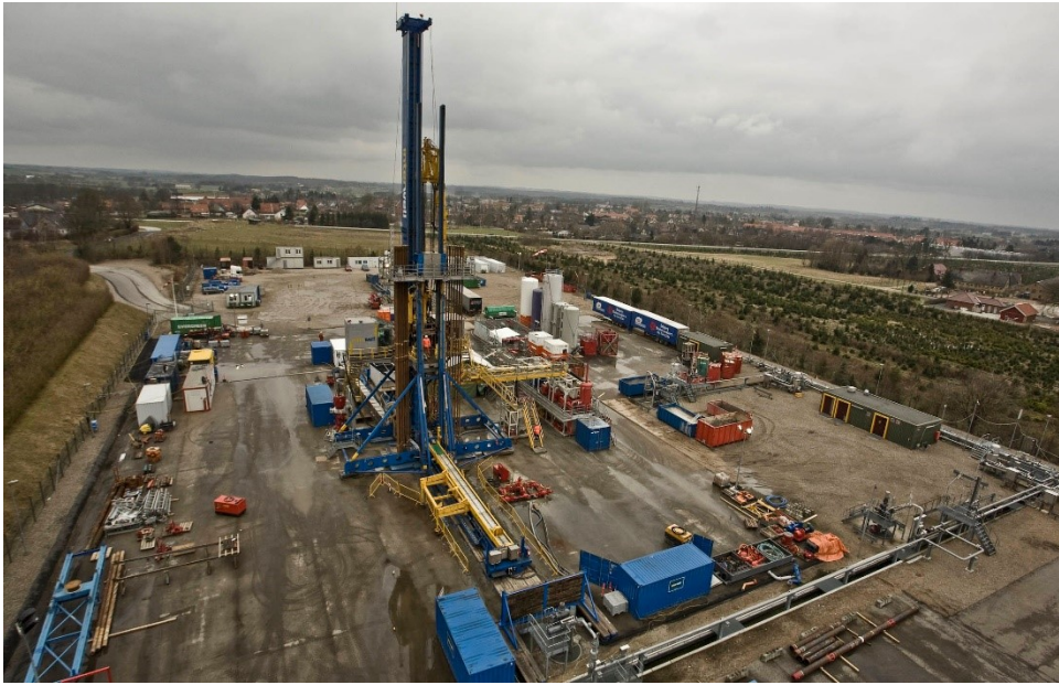
Figure 0-32: Drilling operation at injection well pad [9]
