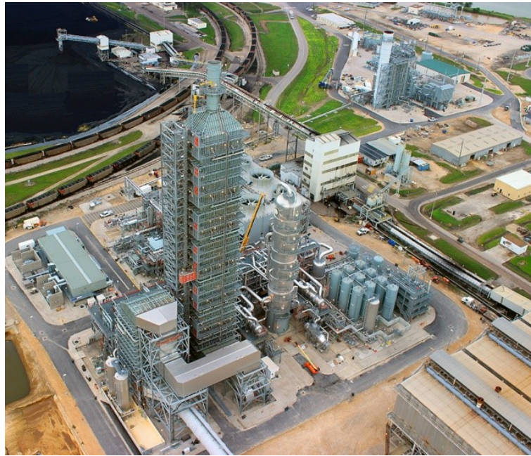
Figure 14. Petra Nova amine CC plant retrofitted to a slip stream of flue gas (equivalent to 240 MWe) from the WA Parish unit 8 coal-fired power plant. [41]
