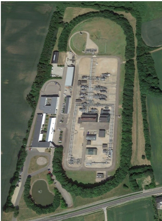
Figure 0-9: Stenlille gas storage [9]
