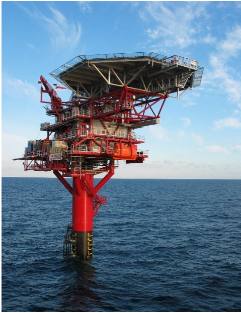
Figure 0-28: Unmanned wellhead platform [20]
