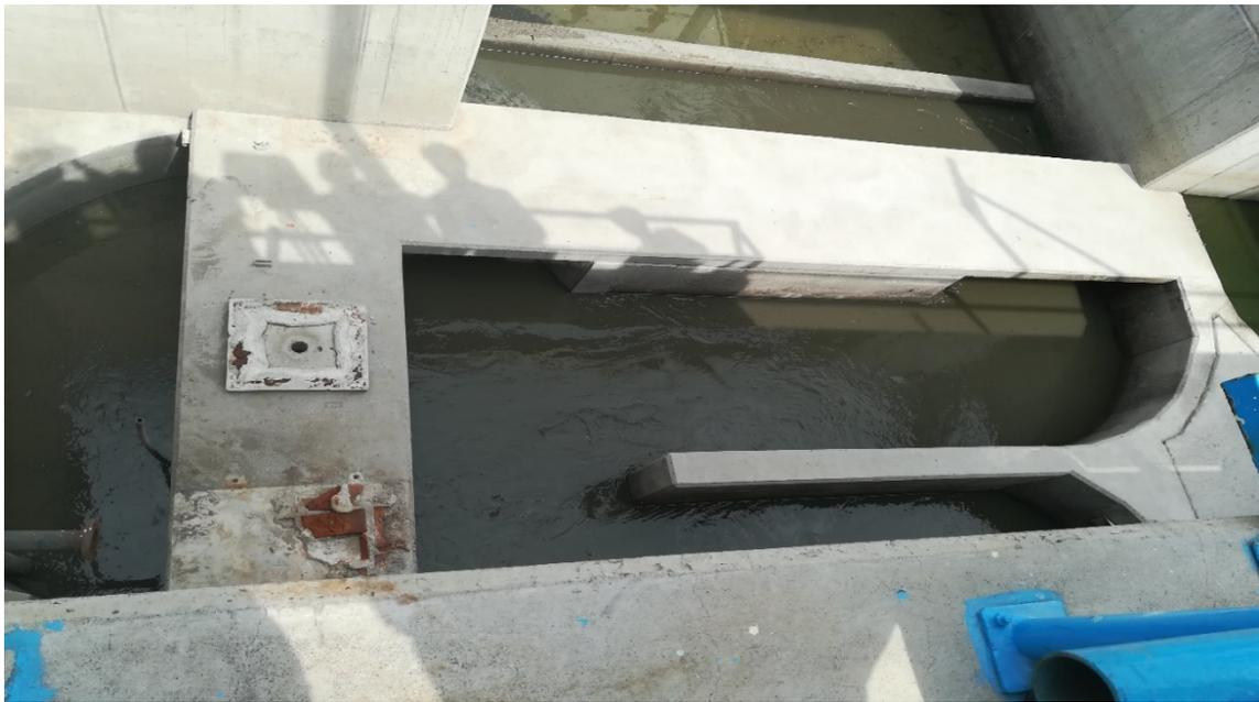
**Figure 6. Structure of the vortex degritter**
