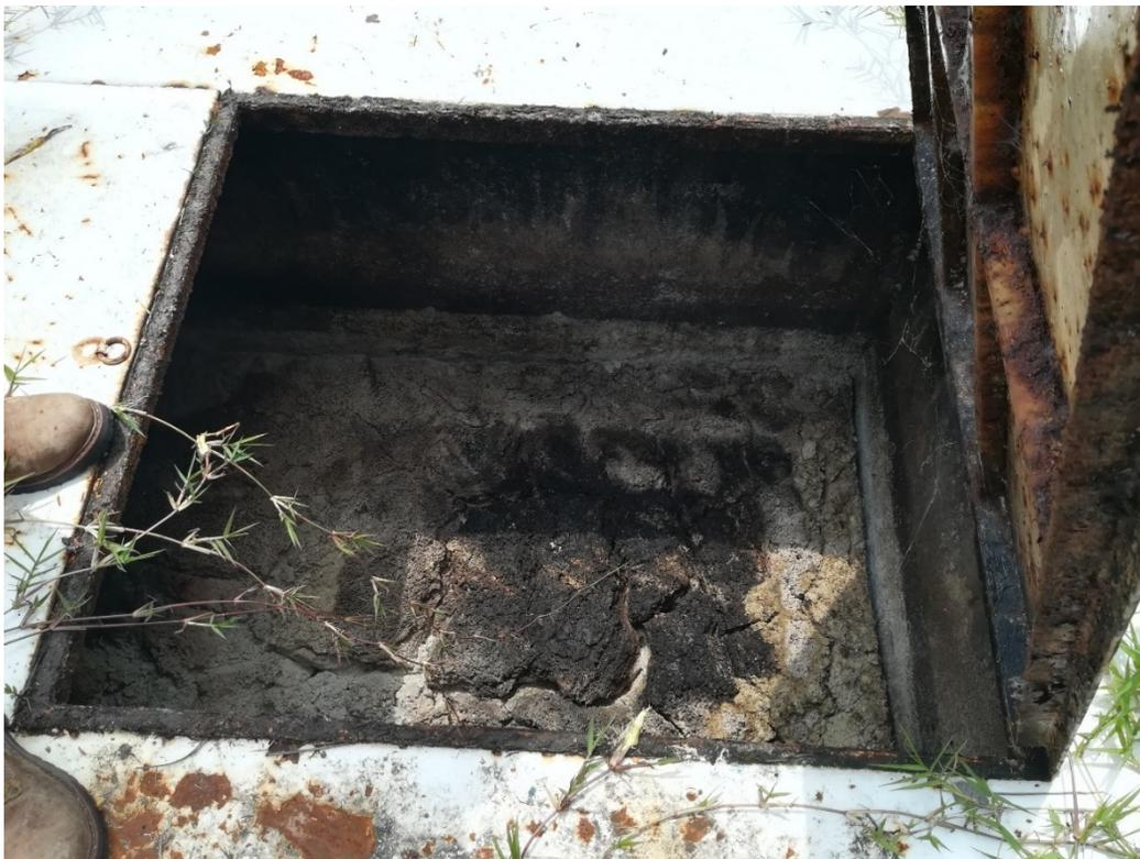
**Figure 36. FOGs accumulation content inside the grease traps**
