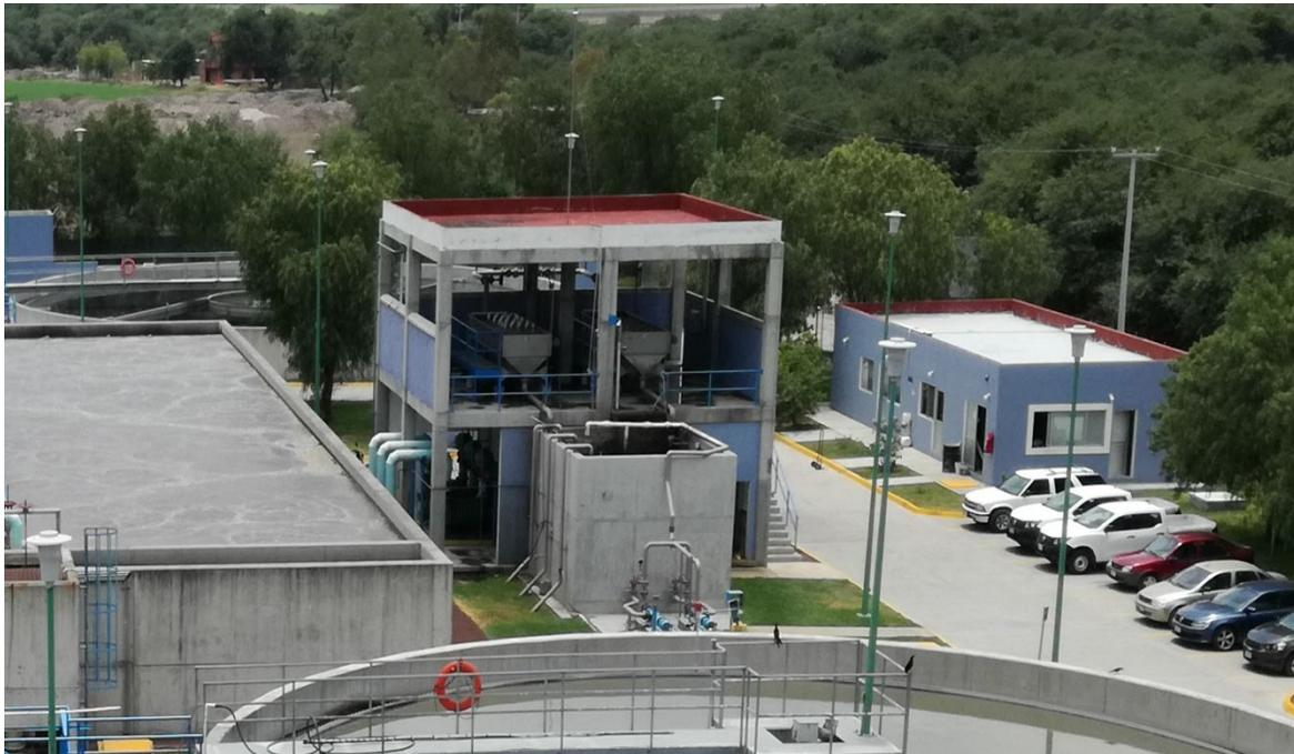
**Figure 14. Thickener and sludge pumping station just up-stream anaerobic digester**
