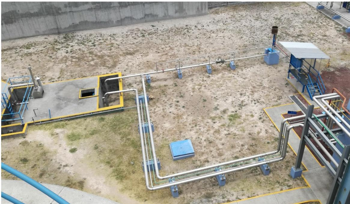
**Figure 13. Biogas burning system**
