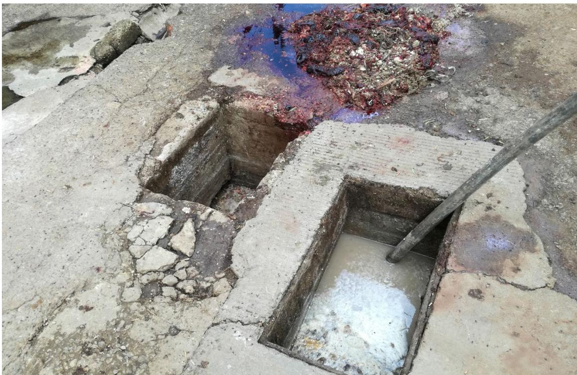
**Figure 27. Grease traps in the slaughterhouse**
