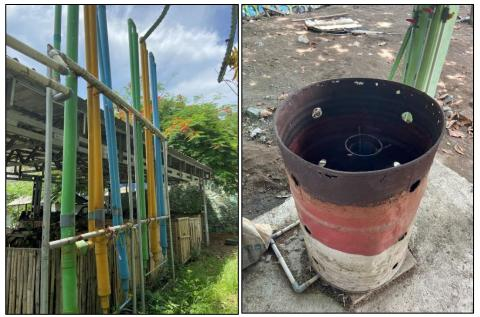
Illustration 4 – Methane capture and gas venting at Kebon Kongok landfill. Photo credit: Viegand Maagoe.
