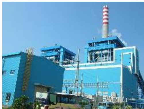
Cilacap Expansion 1 Coal Power Plant in Central Jawa (Ref. 14)
