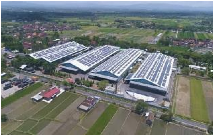
PT Aqua Danone Rooftop PV at Klaten, Central Jawa (Ref. 12)
