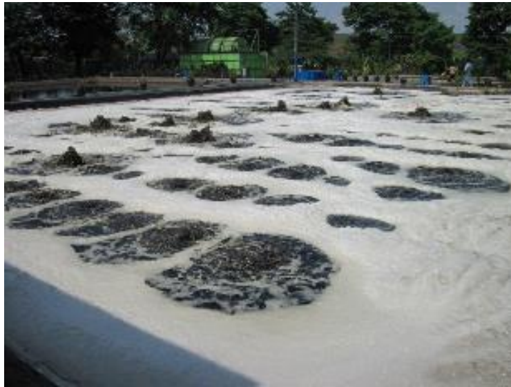
Leachate collection and treatment pond at Bantar Gebang Landfill gas power plant. (ref. 8)
