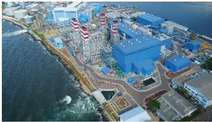
Jawa 2 CCGT Power Plant at North Jakarta (Ref. 5)
