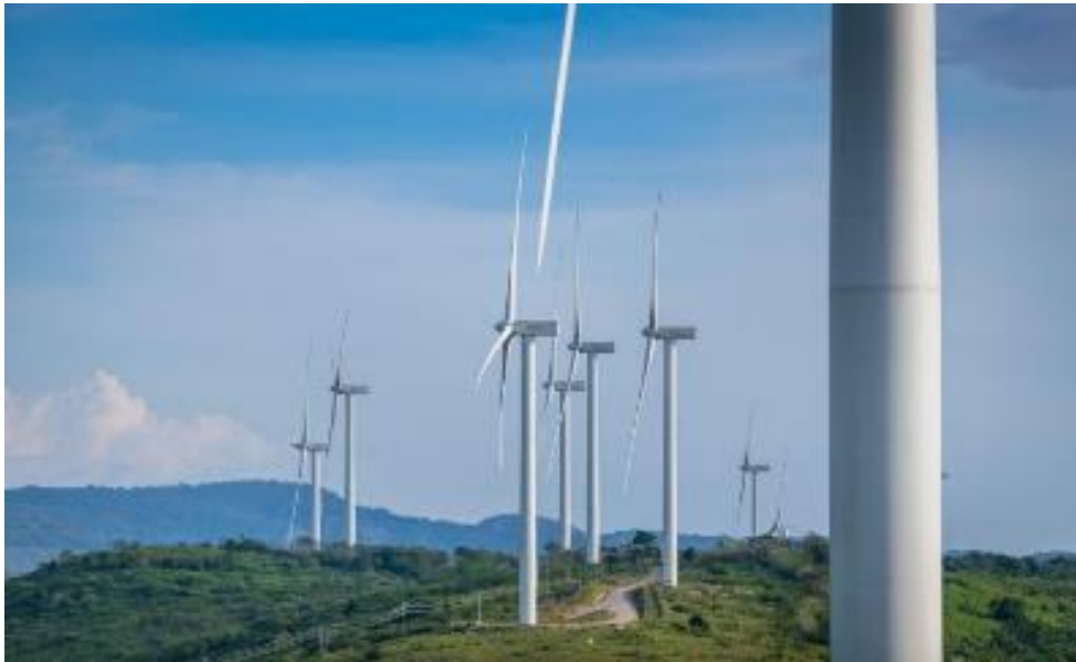
Sidrap 1 Wind Power Plant at Sidrap, South Sulawesi (Ref. 19)
