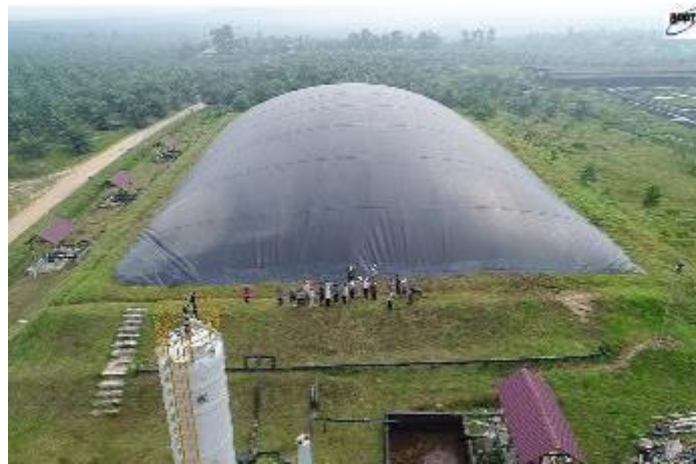
Teratam Biogas Power Plant (covered lagoon type) at Kampar, Riau (ref. 13)
