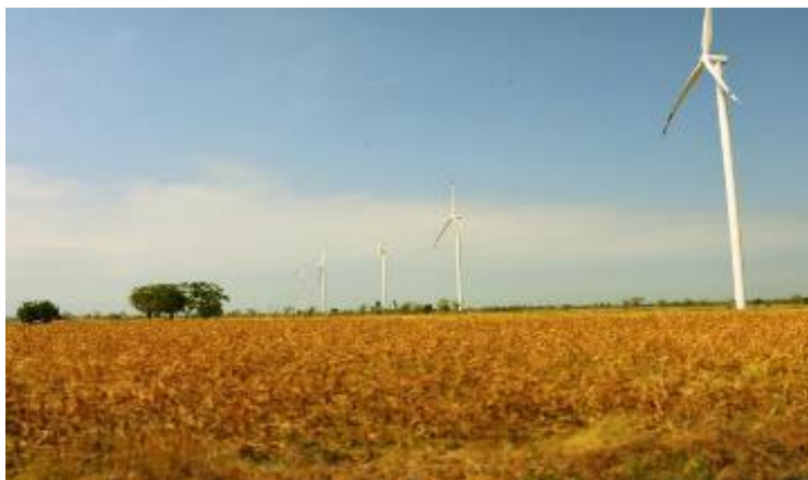
Tolo 1 Wind Power Plant at Jeneponto, South Sulawesi (Ref. 18)
