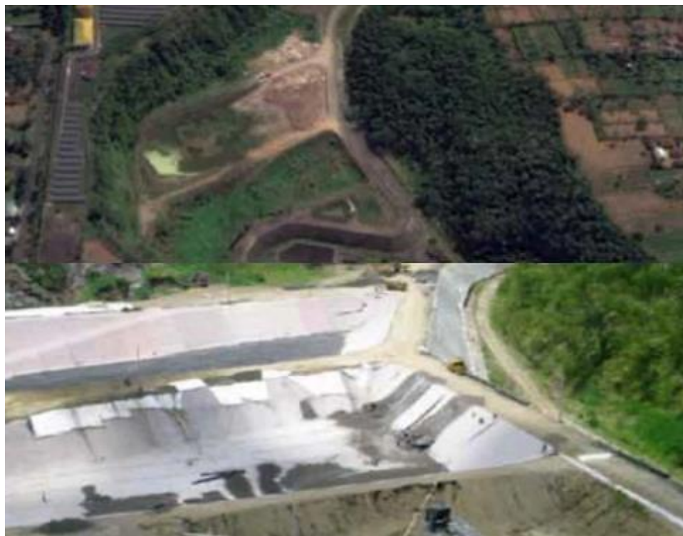
The first sanitary landfill in Indonesia at Bangli, Bali (Source: MEMR (2020), Waste to Energy Guidebook).
