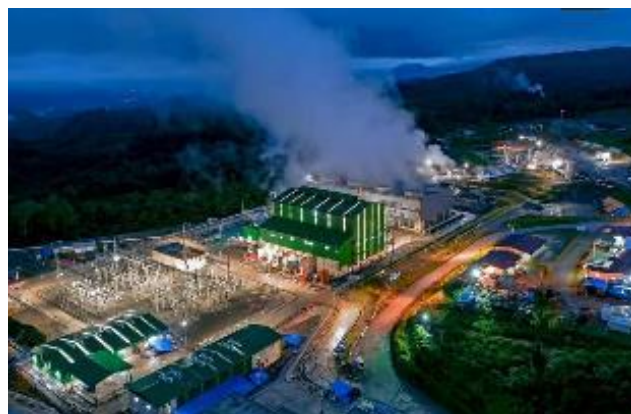
Muara Laboh Geothermal Power Plant (Ref. 14)
