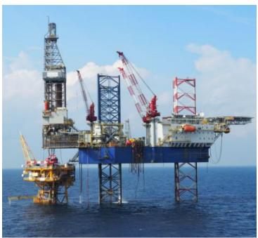
Figure 3.4 Typical Jack-Up Rig
