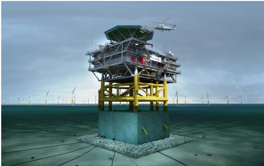
**Figure 3-7 Substation installed with a hybrid foundation.**
