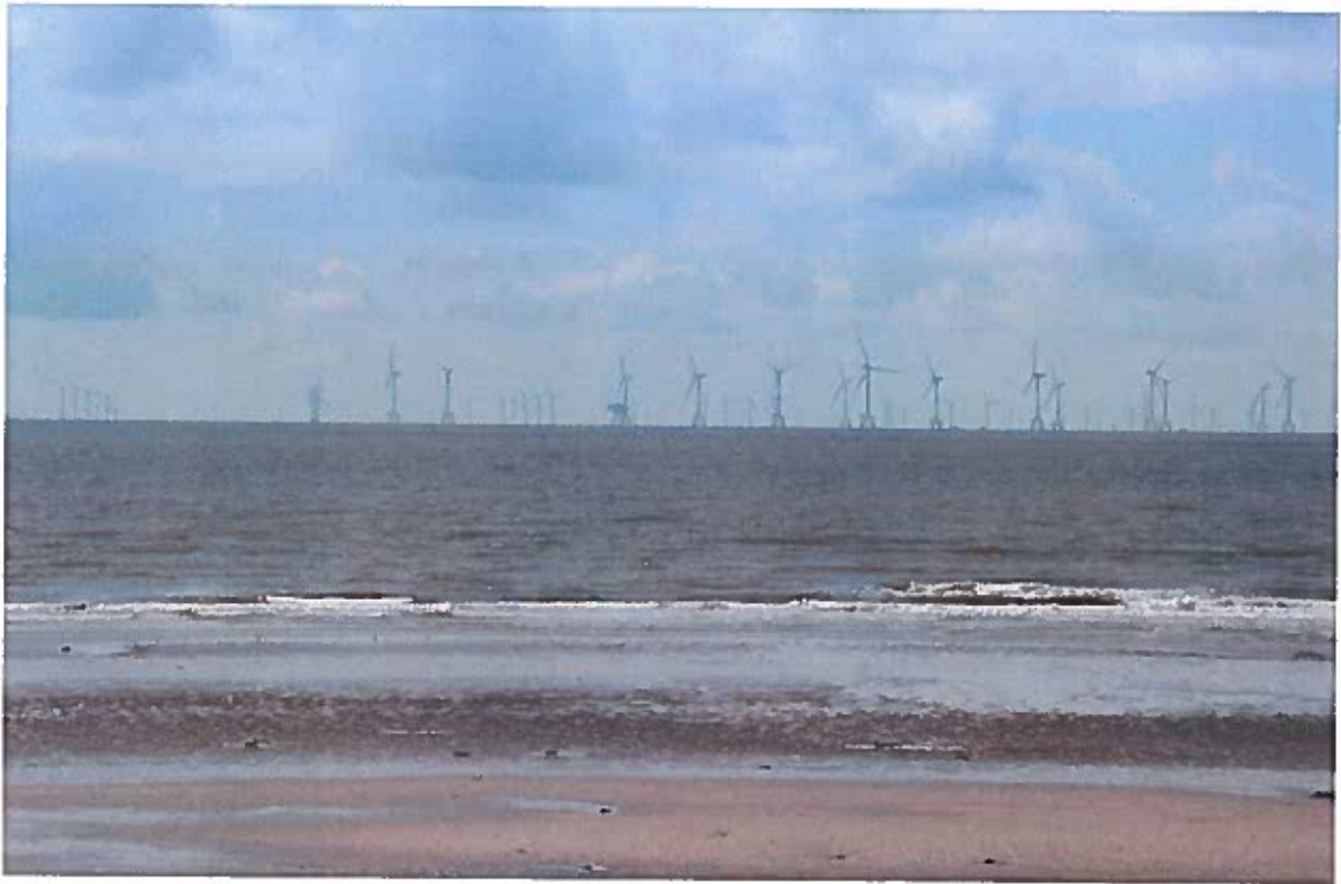
Figure 10. Ormonde (foreground) and Walney (background) wind facilities photographed from Walney Island (Viewpoint V1 in Figure 1), approximately 9.5 km (5.9 mi) from the closest turbine in the Ormonde facility and 17.0 km (10.6 mi) from the closest turbine in the Walney facility. Ormonde turbines are mounted on quadruped structures. An offshore substation is at center left. Equivalent 35-mm focal length = 157 mm.
