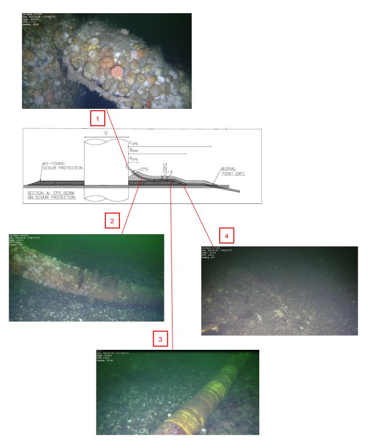
Figure 1: Monopile, cable protection system and scour protection in Anholt Offshore Windfarm (ROV pictures)
