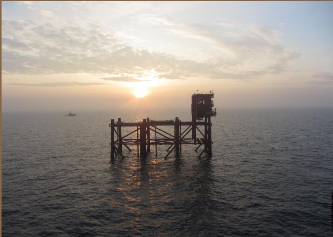
Jacket with wellhead module in the Hejre Field, June 2014.
