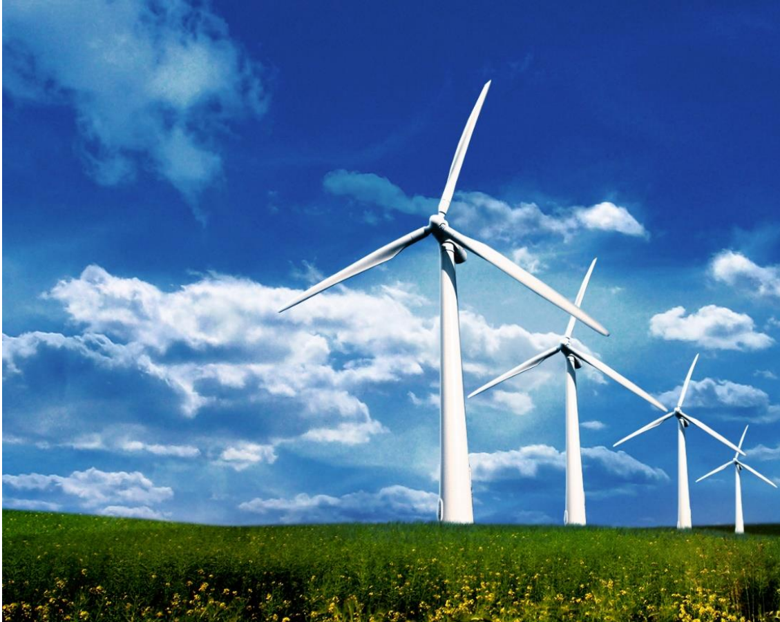
Figure 14 Four Vestas 3 MW wind turbines
